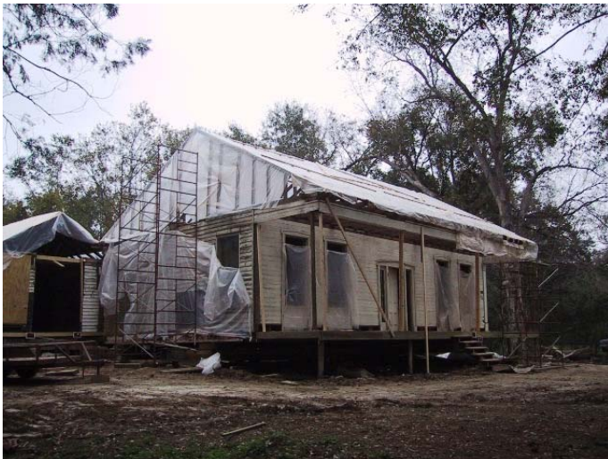
Reconstruction begins with the installation of the roof and ceiling on the front porch (note detail at right) November 2004
