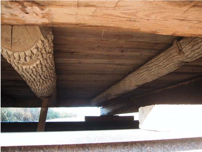
Log floor joists support the older section of the house
